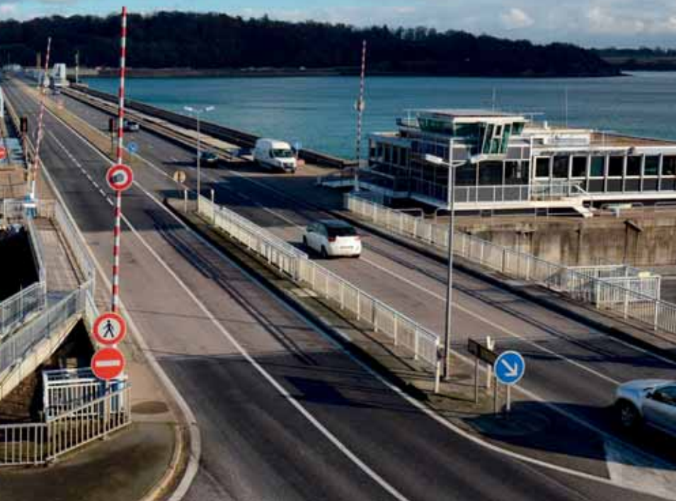
La Rance tidal power station, Brittany, France
