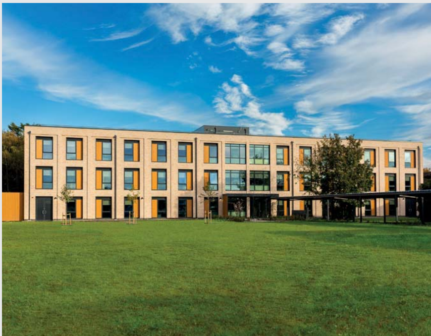
Reds10's award-winning Imjin Barracks in Gloucestershire is made using MMC
