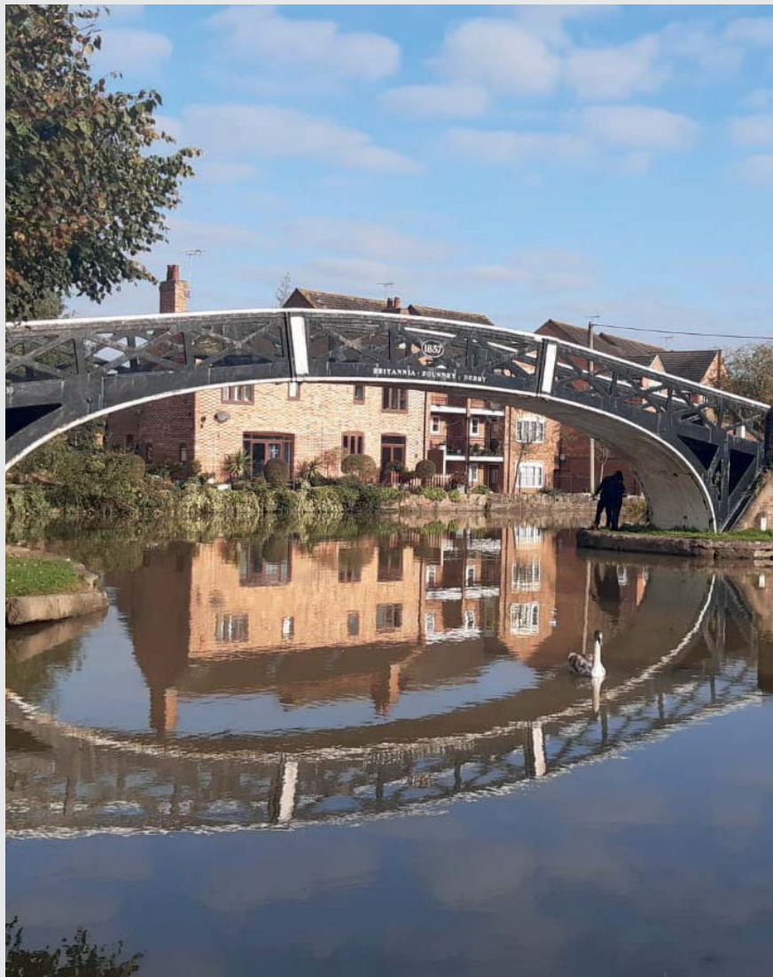
The Grand Union Canal is among the options to transfer water to the south-east
