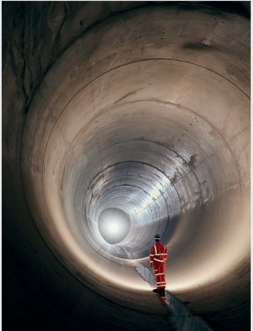
Inside the Thames Tideway Tunnel, which opened earlier this year
